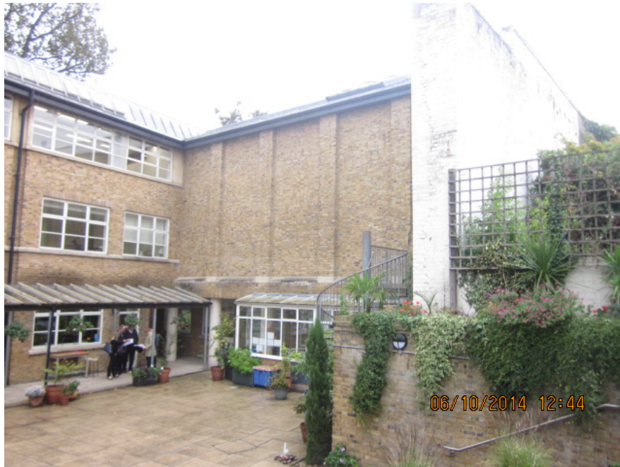
View of Grosvenor building
