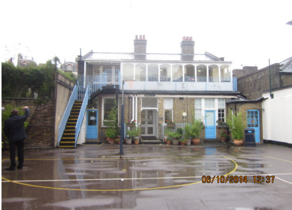
View of Northern elevation of Morison Building
